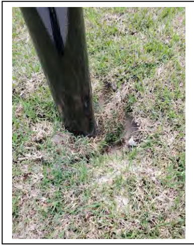
Hole at base of streetlight in the ReCHARGE parking lot.
