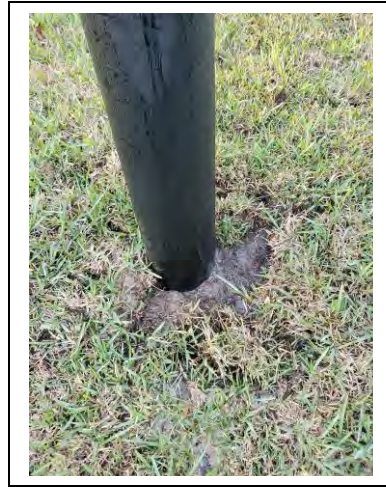
Hole at base of streetlight in the ReCHARGE parking lot.
