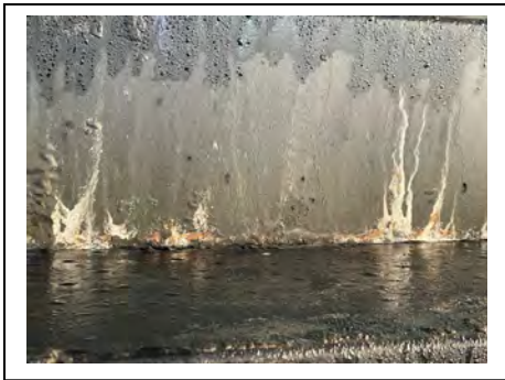
BEFORE BOTTOM OF STAIRS
