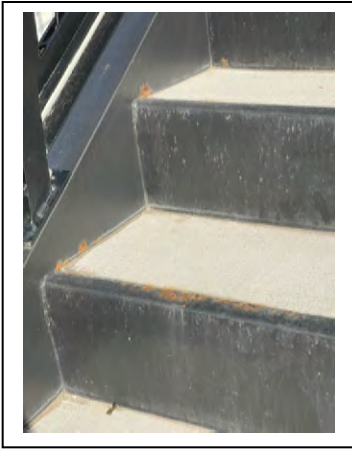
BEFORE TOP OF STAIRS
