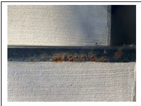
BEFORE TOP OF STAIRS
