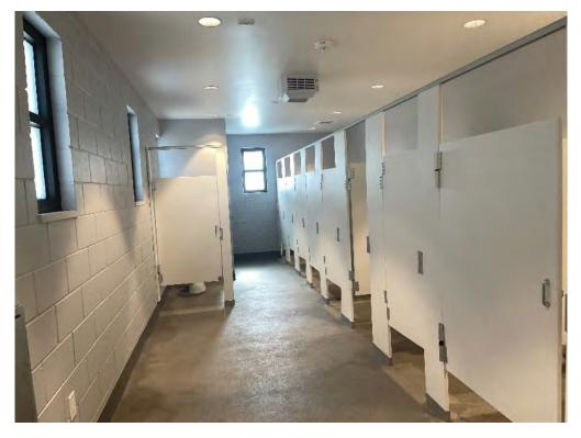
Restrooms have sealed concrete floor and painted CMU walls. Refurbishment includes toilet partitions, fixtures and painting.
